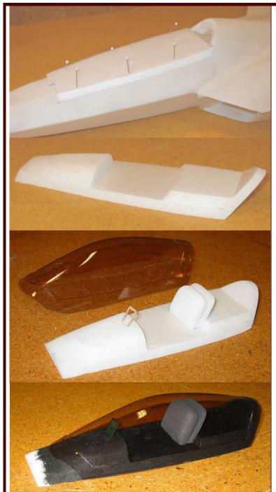
**14.** Next build the canopy. Begin by cutting all the beveled edges on the canopy base parts as specified on the plans. Pin the canopy base to the model and sand the edges so they're flush with the fuselage sides.
